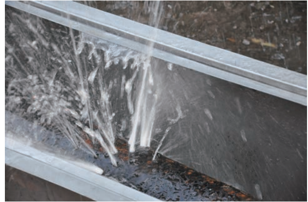
Fig. 8 Photograph of outlet flow at location D of screen No. 2 after cleanup
