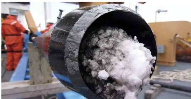
Fig. 1. Hydrate blocking submarine pipeline.
