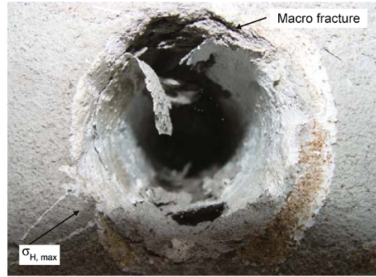
Fig. 13 Damaged zone around borehole before critical condition
