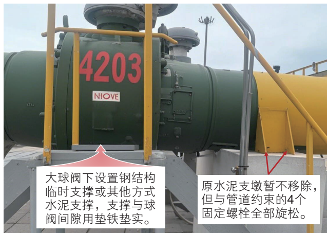
图 10 现场工艺优化方案实物图 Fig. 10 Physical diagram of the on-site process optimization scheme
